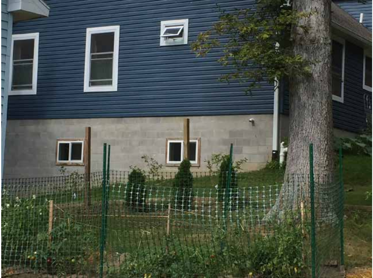
The tops of the 4x4 are at 6 ft. The windows in the block foundation are in the cellar of neighboring property.
